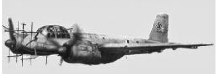
Luftwaffe Ju 88 fighter with radar equipment mounted on the nose
