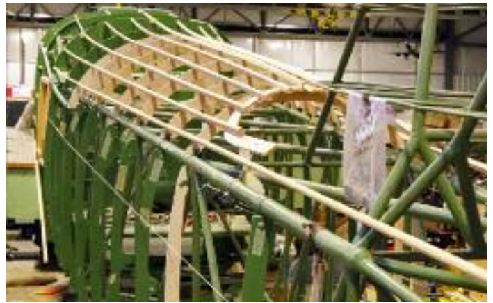
The Anson's fuselage is made up of a steel tube framework that supports wooden stringers and formers. Eventually these will be covered with fabric.
